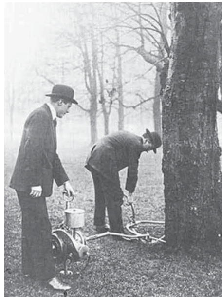
Fig. 14. A Sector saw during site tests in 1917 ( www.solhem9.se )
